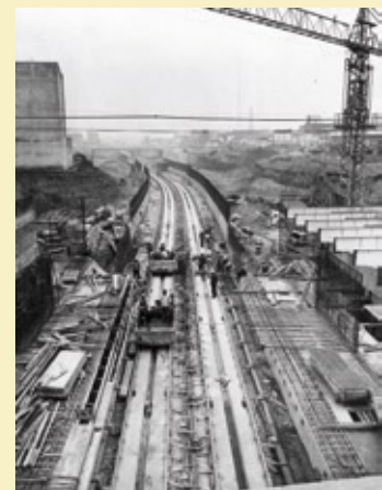
Construction of the first section of Line 2.
