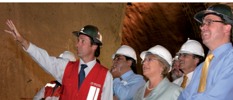
» Presidential visit to the extension works of Line 5.
