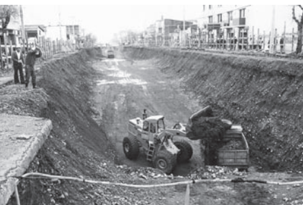
» Works in Alameda for the construction of Line 1.
