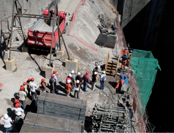
» Close to 2 thousand people visited the Metro extension works during 2008.
