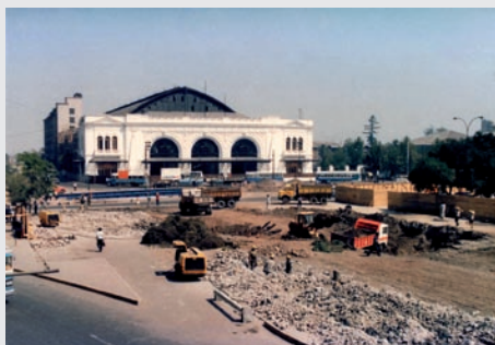
» Construction of Puente Cal y Canto station.
