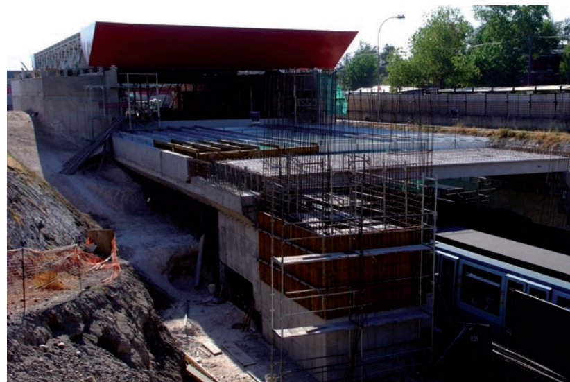
» Works in Pajaritos station.
